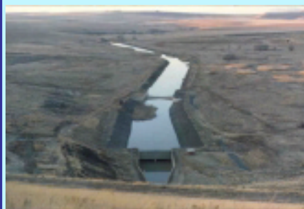
STERKFONTein DAM OUTLET WITH CRUMP WEIR
